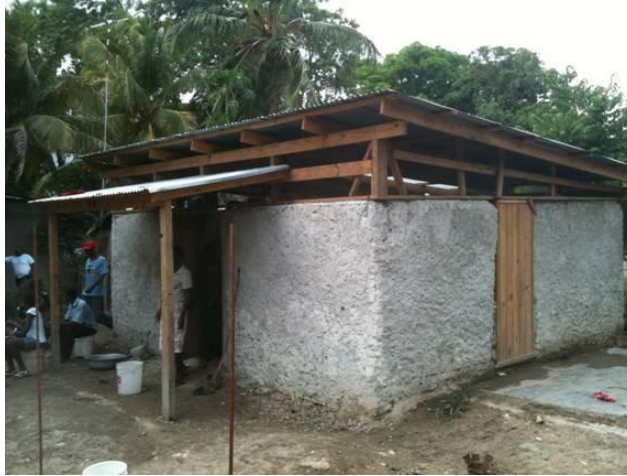
Safe, permanent housing for Haitians
